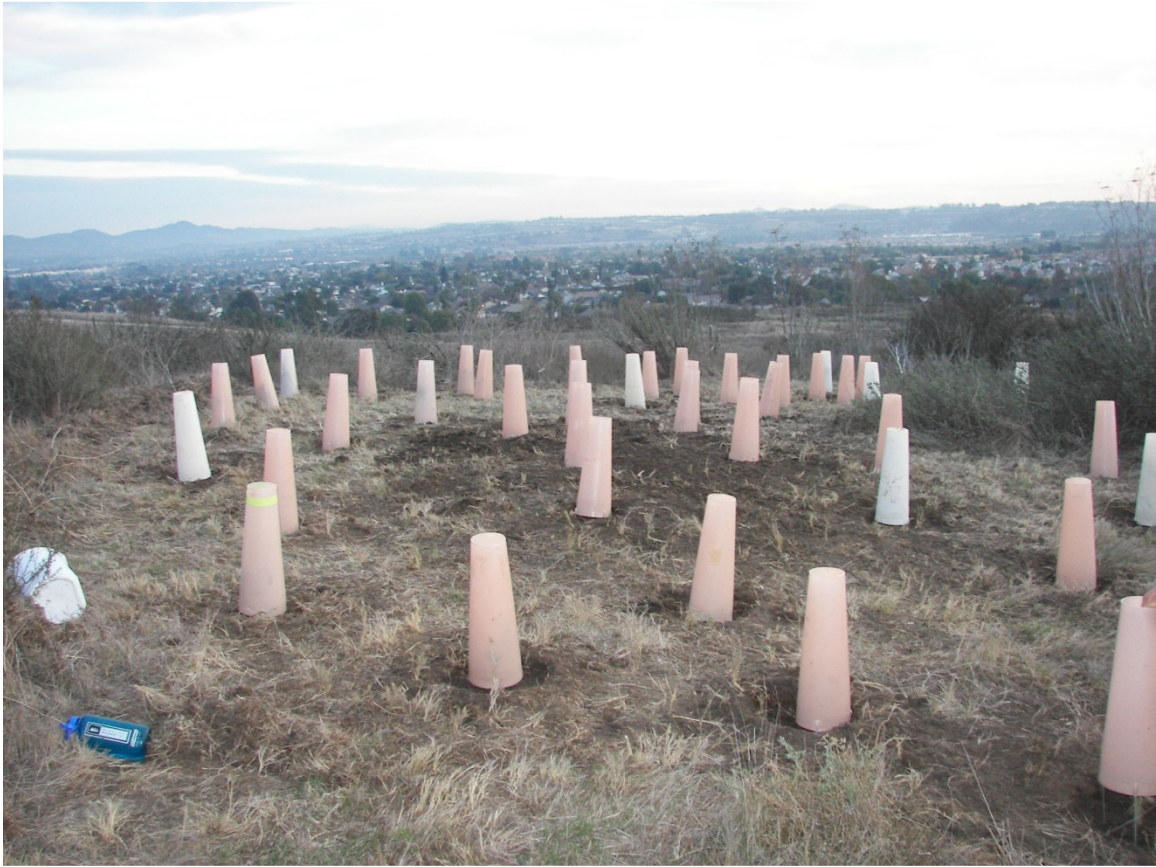
Photograph 2: 0.05-acre restoration area after plant band installation.
